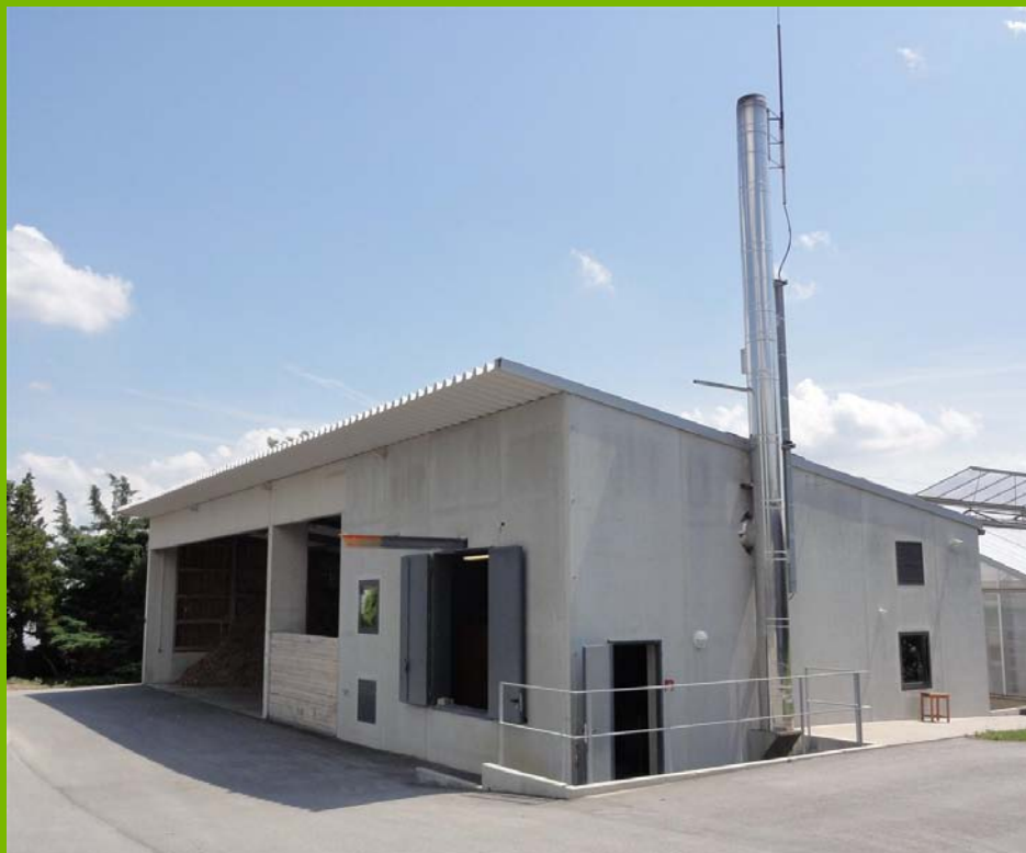
Biomass heat plant at the University of Applied Sciences, Weihenstephan, built in 2008. 850 KW thermal, 5000 m 3 forest residues replace 300 000 l heating oil every year and generates regional income. Total investment about 1 M AUD, calculated payback period about 5 years.
